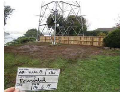
Tower (after) with foundations completed and wooden fence replacement, prior to grass regrowth.
