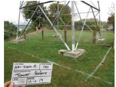
Tower (before) – note steel wire fence through middle of tower.
